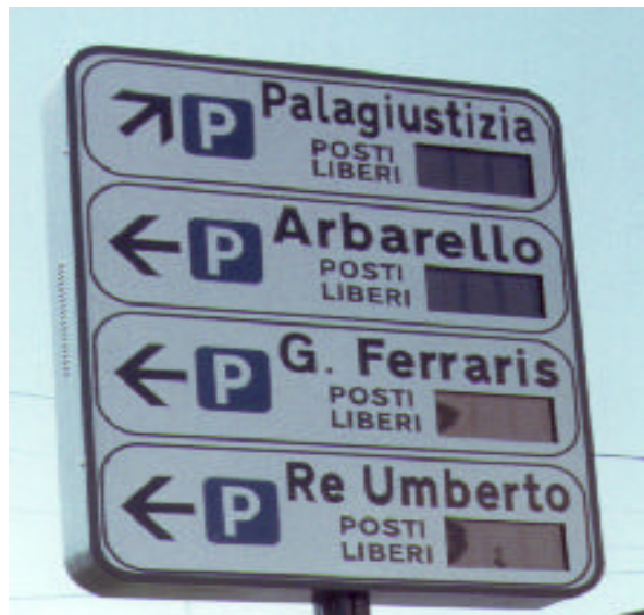
Figure 23: Variable Direction Sign panel adopted in Turin for Parking Guidance
